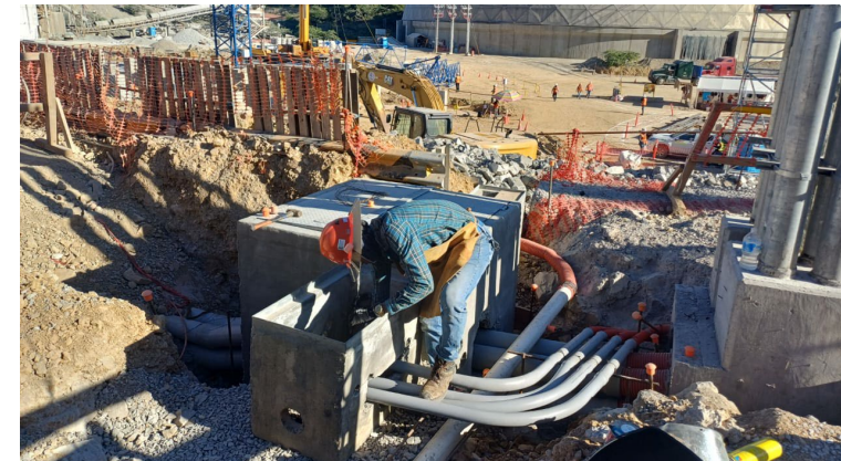
Installation of communication and electrical conduits
