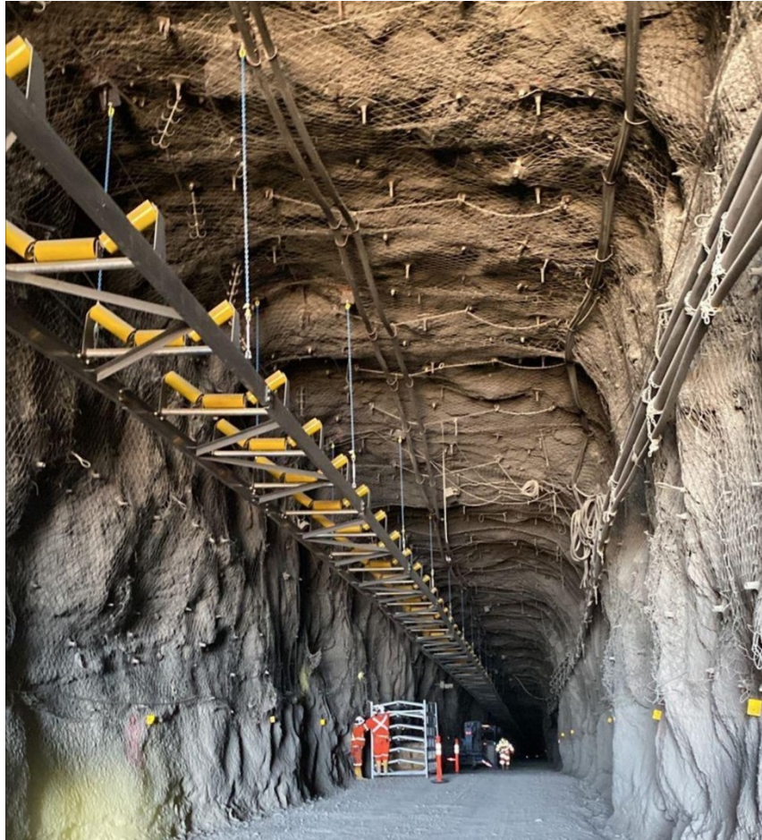
Figure 1: Following completion of the Guajes Tunnel in December 2023, significant progress has been made on the seven-kilometre conveyor with 78% of conveyor tables installed
