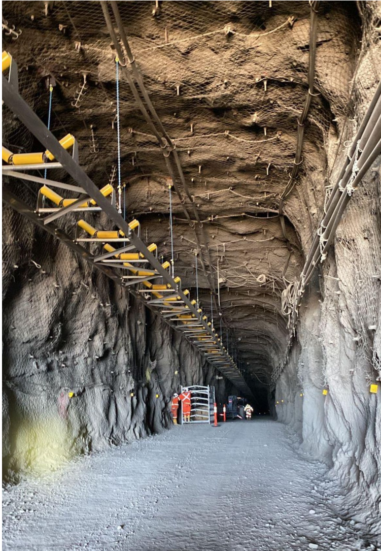
Conveyor table installation
