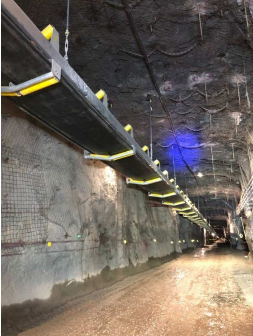
Conveyor belt installation
