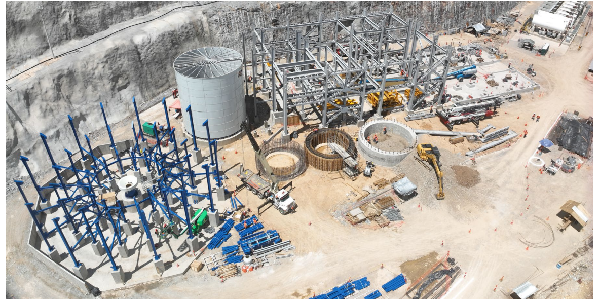
Steel erection and assembly for paste plant
