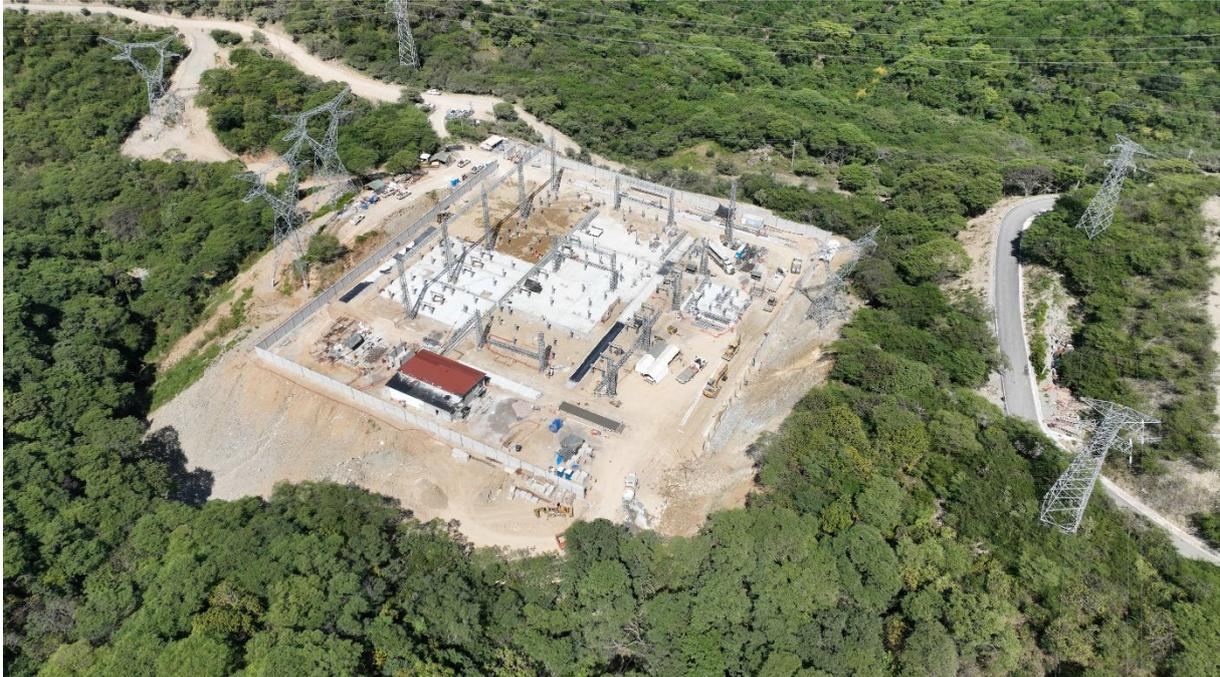
Figure 5: The 230 kV substation is substantially complete with main transformers in place
