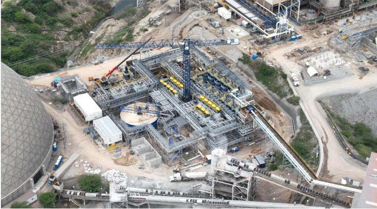
Figure 3: Construction of the water treatment plant is ongoing, with detox tanks for the first phase of water testing installed during the quarter
