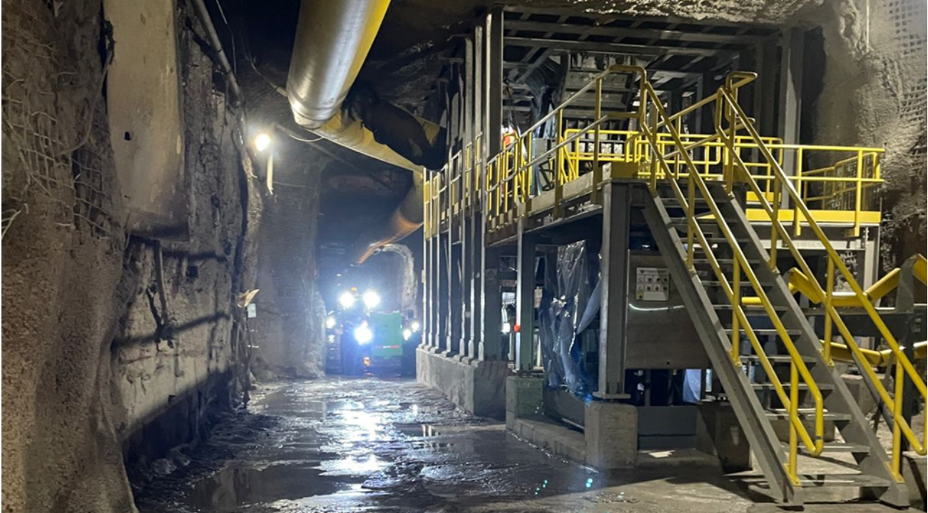
Figure 1: Ore bins feed chutes have been assembled at the 690 level
