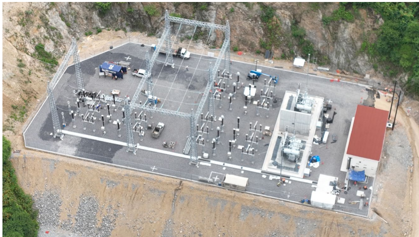
230 kV substation substantially complete
