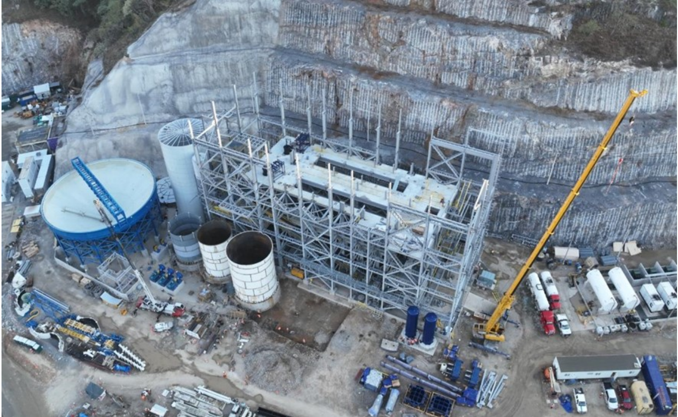
Figure 4: Work progressed on the paste plant during the quarter, including continued erection of the binder silo, thickener, and building steel.
