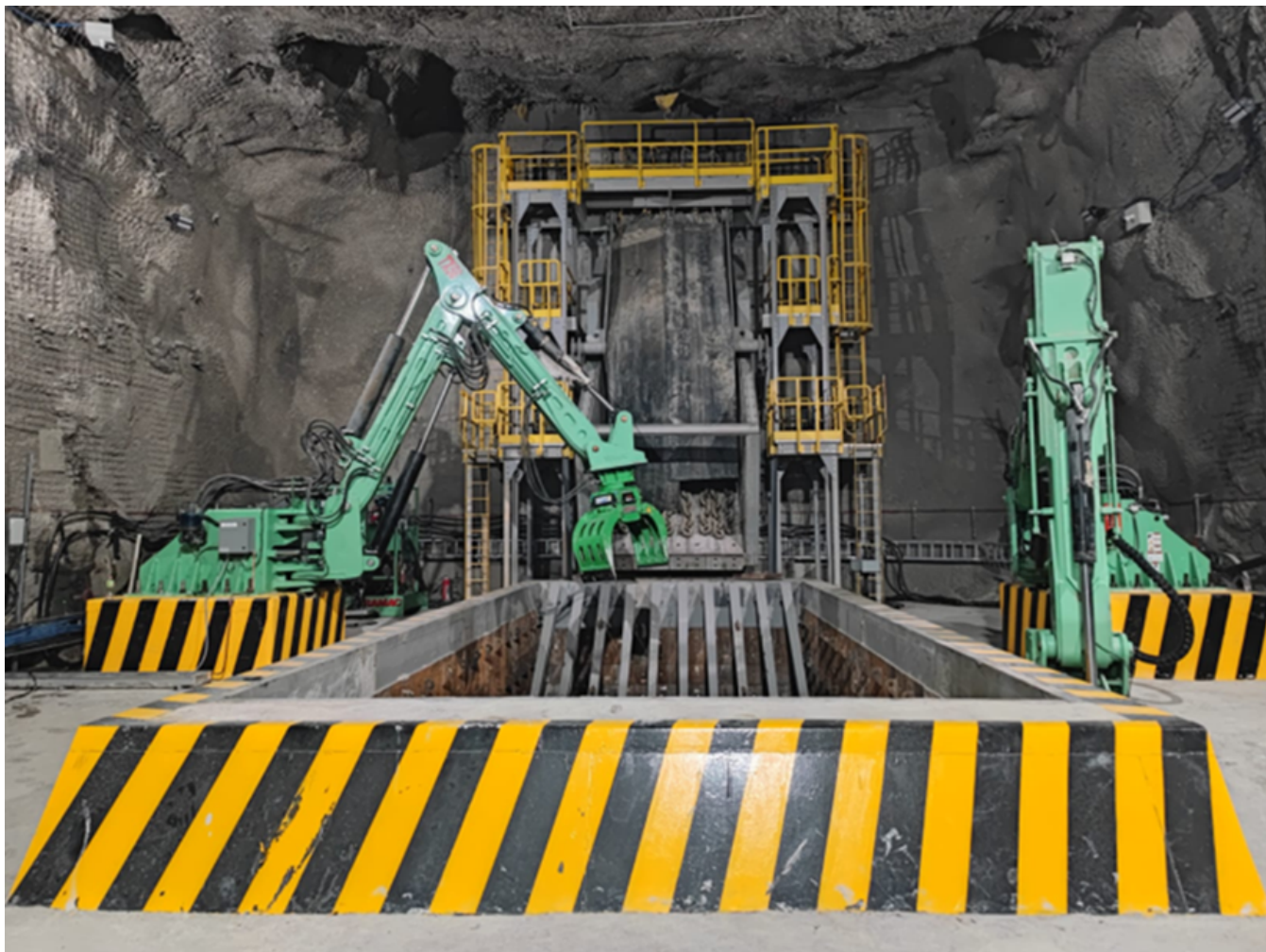
Figure 1: Rock breaker #1 and the grizzly chute have been installed and commissioned.
