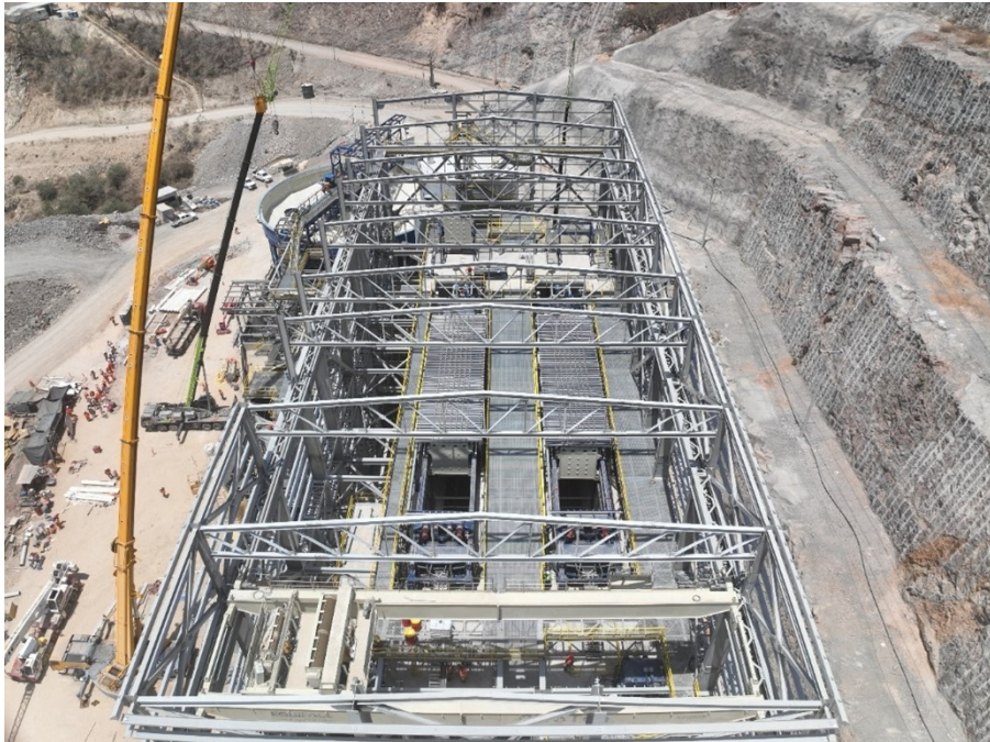
Figure 3: Paste plant filter installation.
