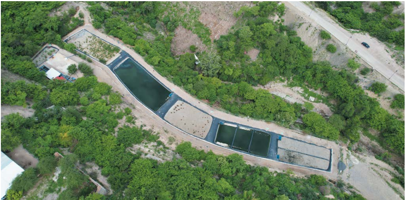
Constructed Wetland Wastewater Treatment System serving the El Limón community
