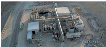
Paso Limonero Wastewater Treatment Plant Infrastructure
