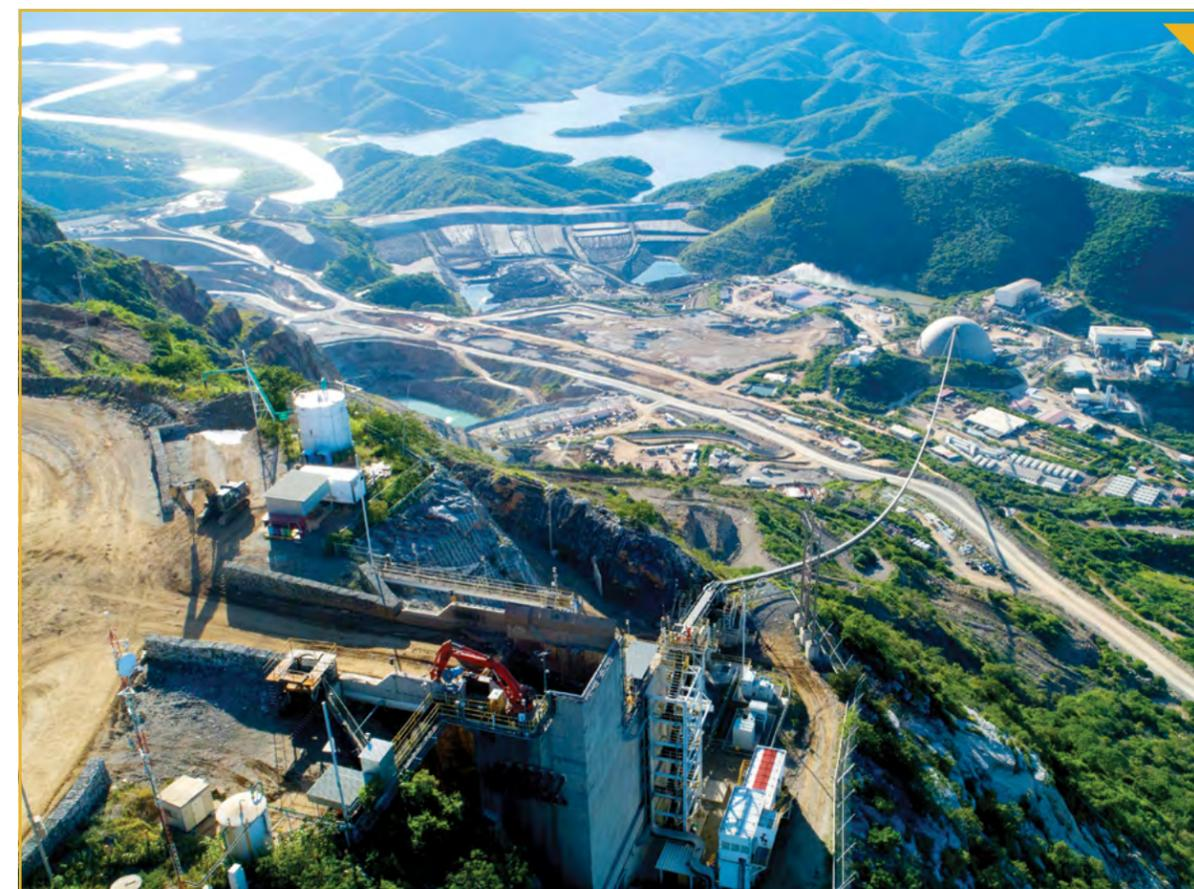
Currently, our main energy consumption sources and emissions derive from electricity usage at the ELG Mine Complex processing facilities and diesel consumption by mobile equipment. A full 100% of our electricity is supplied by the Mexican power grid operated by the Federal Electricity Commission (CFE). Backup diesel generators are also in place at processing facilities and our residential camp to ensure uninterrupted operations.
