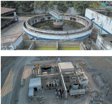
Paso Limonero Wastewater Treatment Plant Infrastructure
