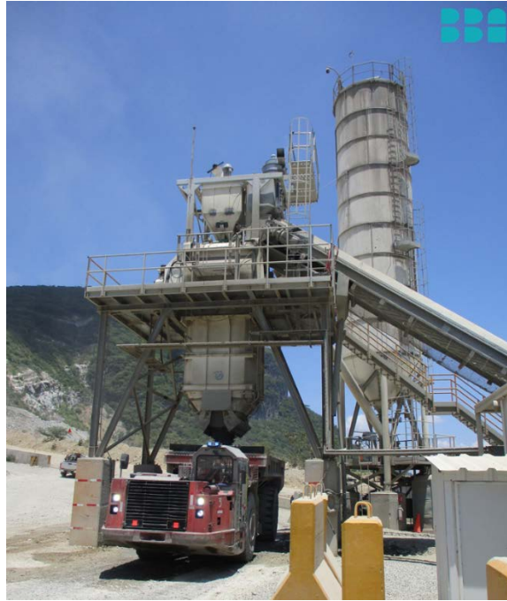
Figure 16-62: Truck Loading Backfill
