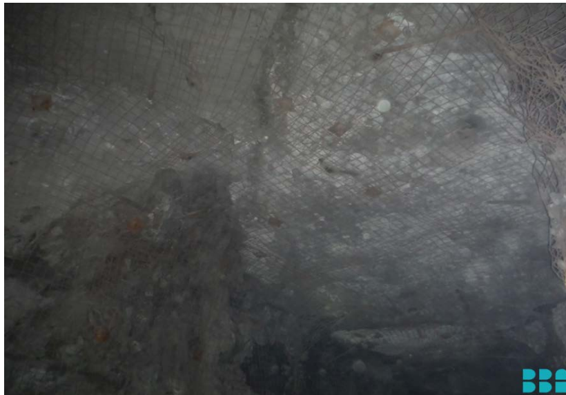
Figure 16-65: Panel Under Backfill
