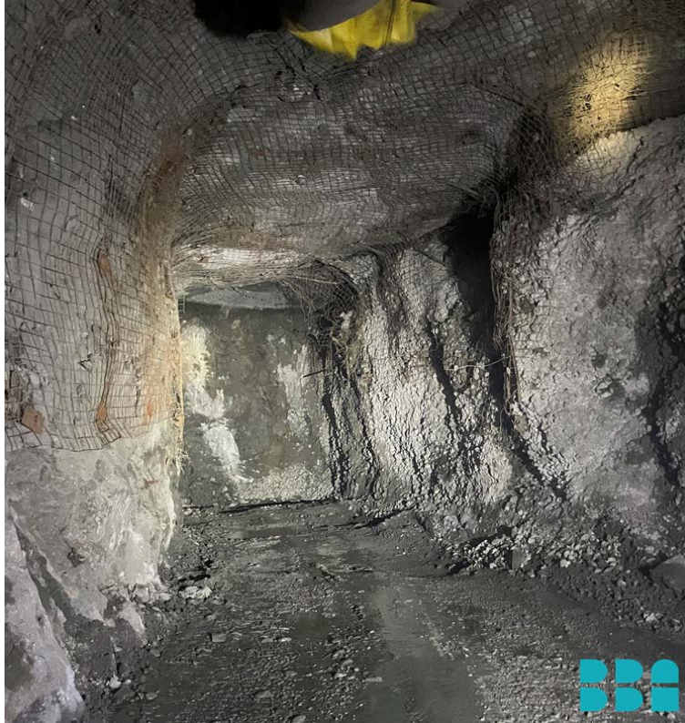
Figure 16-64: Panel Beside Backfill Panel
