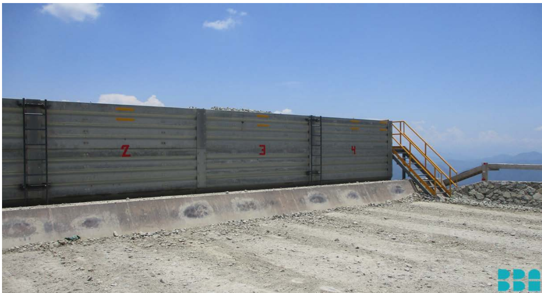
Figure 16-57: Backfill Plant Aggregate Bins
