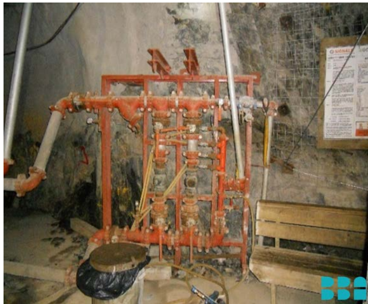
Figure 16-75: Typical Pressure Relief Arrangement
