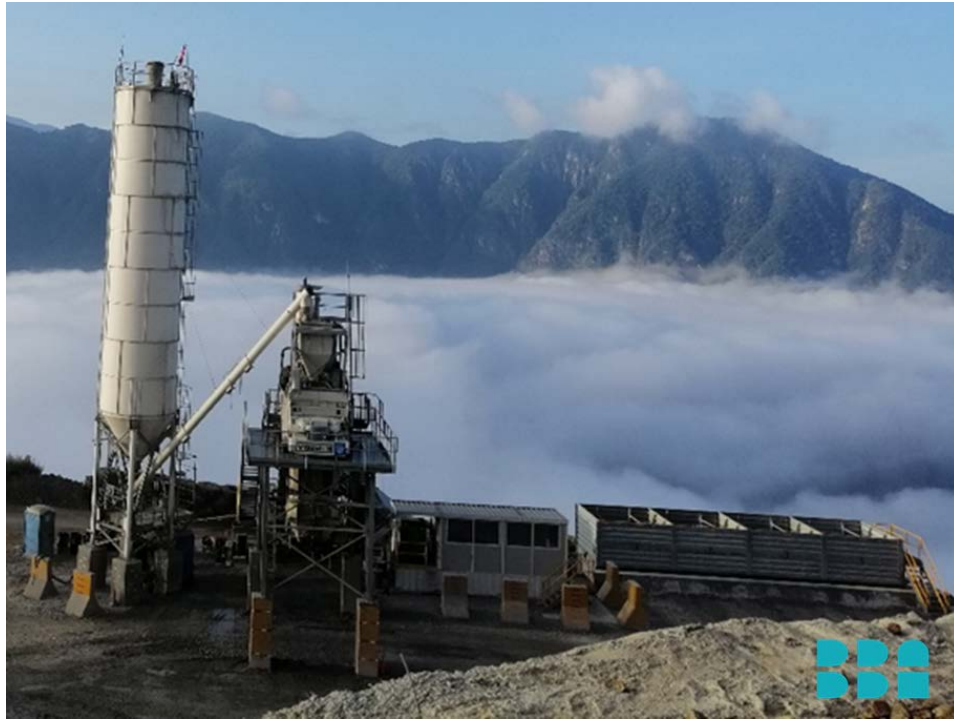
Figure 16-56: CRF Plant and Portal 2
