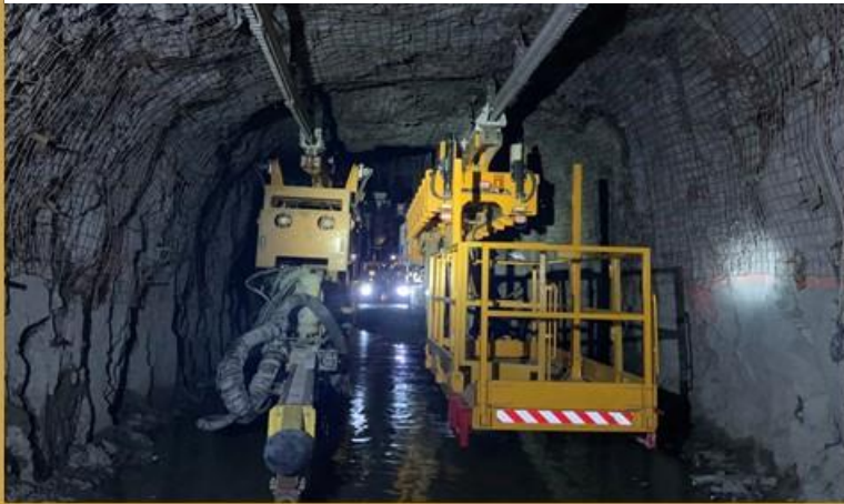
Moving equipment with 2 lane traffic
