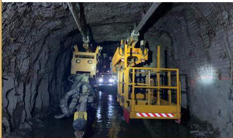
Moving equipment with 2 lane traffic
