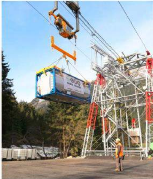
Figure 24-17: Ropeway Elevated Cable Crane System (Courtesy of LCS)
