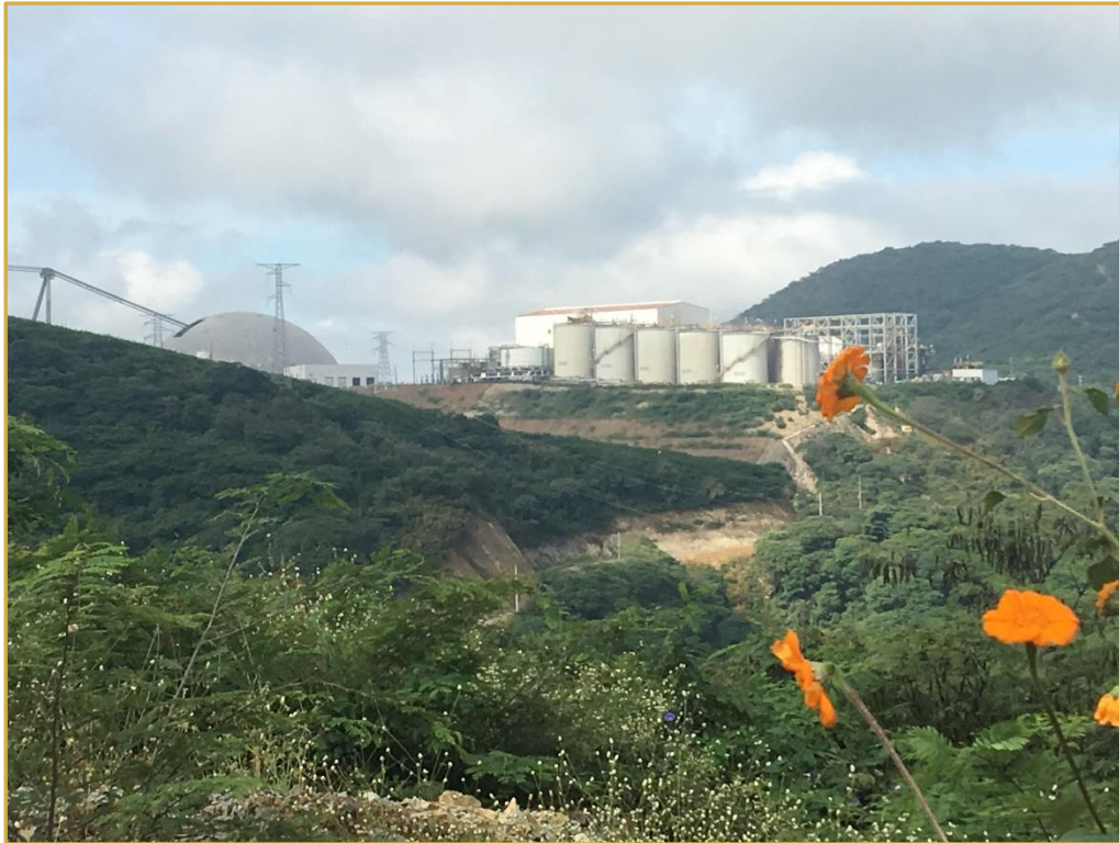
ELG Processing Facilities with RopeCon and Stockpile Dome on the left
