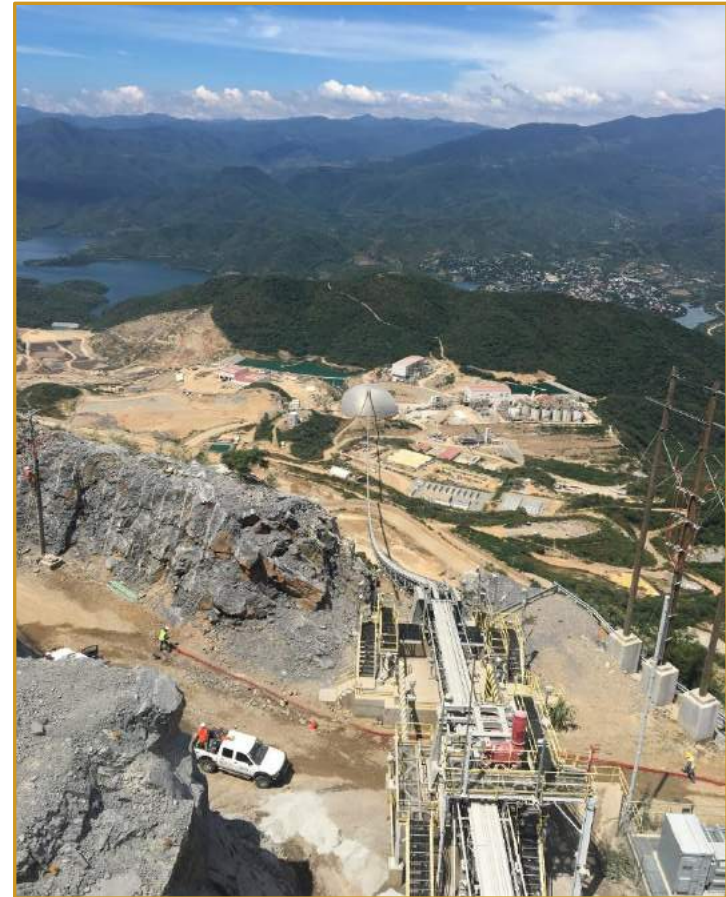
View from the Top of the RopeCon at El Limon Pit
