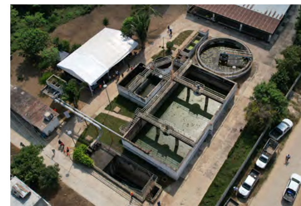
Paso Limonero Wastewater Treatment Plant, Acapulco
