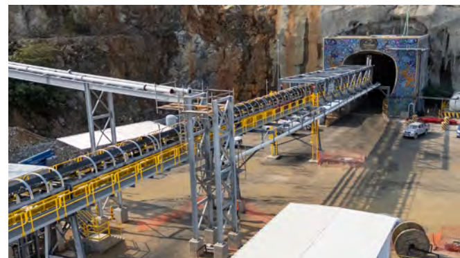
The Guajes Tunnel Conveyor
