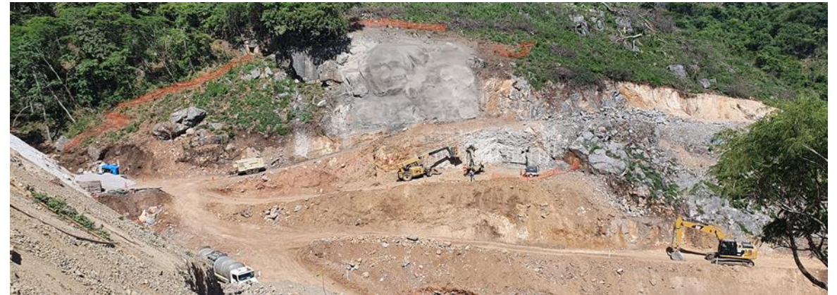
Prep of South Portal Upper well underway
