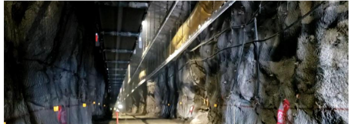
Guajes tunnel has advanced 450 m
