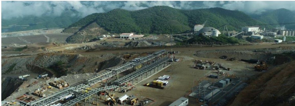
Overhead shot of loadout facility and plant
