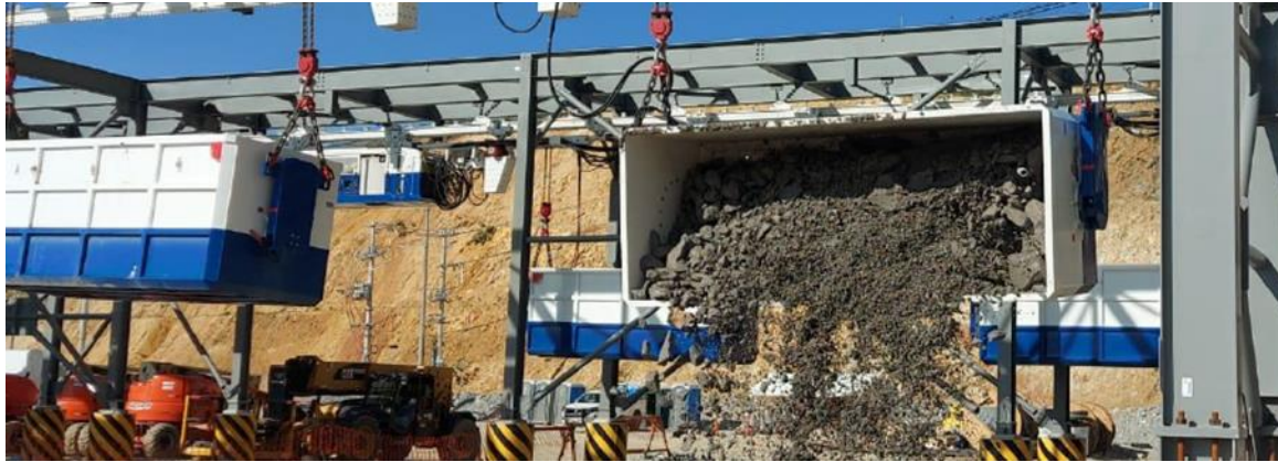
Monorail-based haulage for waste rock
