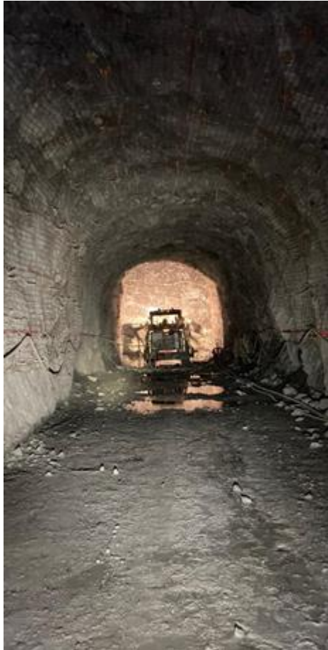
Tunnelling in South Portal Lower
