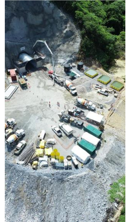
Canopy completion (South Portal Lower)
